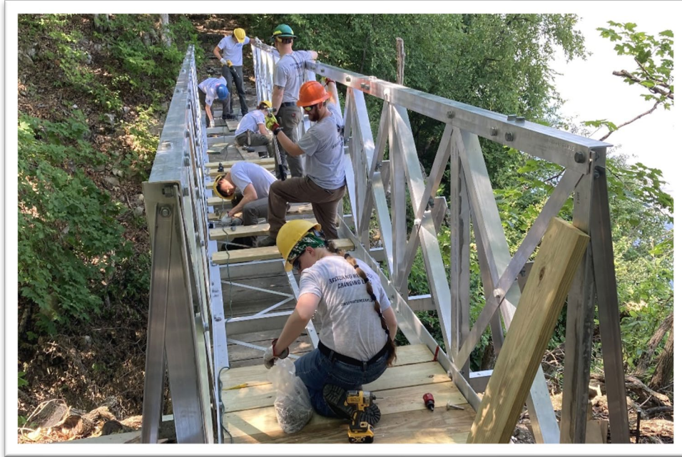
Iowa Crew Building a Bridge, 2024
